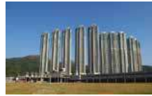
LOHAS PARK RESIDENCE Tseung Kwan, Hong Kong
